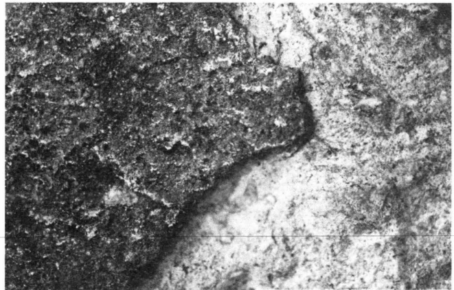
FIGURE 3 Delamination of concrete below carbonated surface.
