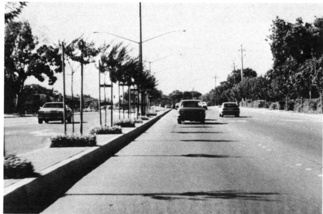
FIGURE 13 A long median nose will result where a left-turn bay is designed to accommodate high off-peak speeds appropriate to major arterial streets or where long queues must be stored during peak periods. Landscaping helps delineate and enhance the visibility of these intersections. A width of at least 6 ft (preferably at least 8 ft), face-to-face of curb, is needed for pedestrian refuge as well as to accommodate landscaping. In this example, the planter boxes contain flowers, which represent a high-maintenance item. Selection of perennial plants will reduce the maintenance cost.
