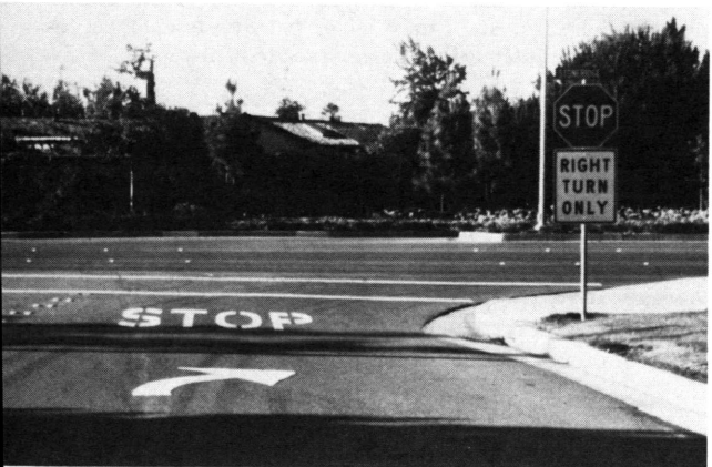
FIGURE 12 Examples of landscaping design to provide good delineation of a median break designed for left-turn egress only. top , driver's view on the approach to the left-turn bay; bottom , view of the median treatment from the intersecting access.
