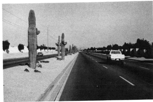
FIGURE 16 US-60/69 in Sun City, Arizona, is an example of medial landscaping using native materials resulting in low maintenance cost and providing good visibility.
