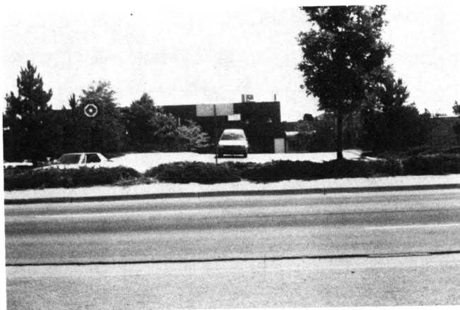
FIGURE 15 This section of US-36 in Boulder, Colorado, was reconstructed with a nontraversable, landscaped median. Movements are now restricted to right turns only. The landscaping adds aesthetics as well as function.
