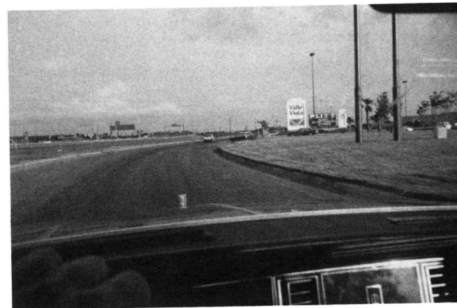
FIGURE 17 Signing must be considered part of the design of intersections that provide access to development. The sign is located on the far side of a divided access drive to a regional shopping center. The problem is compounded by the intersection's location on a horizontal curve to the right. These two elements combine to lead drivers past the ingress drive. Many drivers miss the drive at night and stop in the traffic lane. Of those who stop, most either back up to enter on the ingress side or enter using the egress side of the drive.
