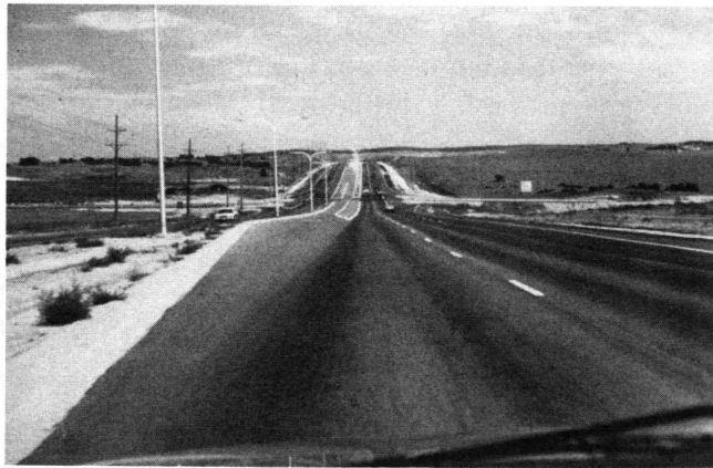
FIGURE 8 When this roadway (Powers Boulevard, Colorado Springs, Colorado) was reconstructed as a multilane major arterial, long dual left-turn lanes (970 ft, including taper) were provided. The bay is currently striped to operate as a single left-turn lane until volumes require a dual left. Such a length will accommodate maneuvers at a 55-mph off-peak speed and ensure availability of maneuver plus storage space when the area fully develops.
