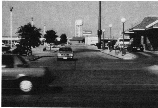
FIGURE 11 Sharing of access will reduce the number of access drives and increase their spacing, or parcels with smaller frontage can be developed given a driveway spacing or corner clearance. In this example, a fast-food restaurant shares access with a 200,000-ft 2 shopping center. The centerline of the access drive is located on the property line. A reciprocal easement runs the length of the restaurant property. This is the only direct access to the restaurant.
