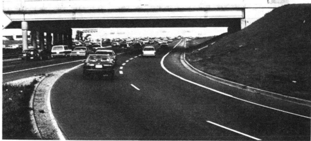
FIGURE 4 Two-lane entrance to freeway from loop ramp (Toronto).
