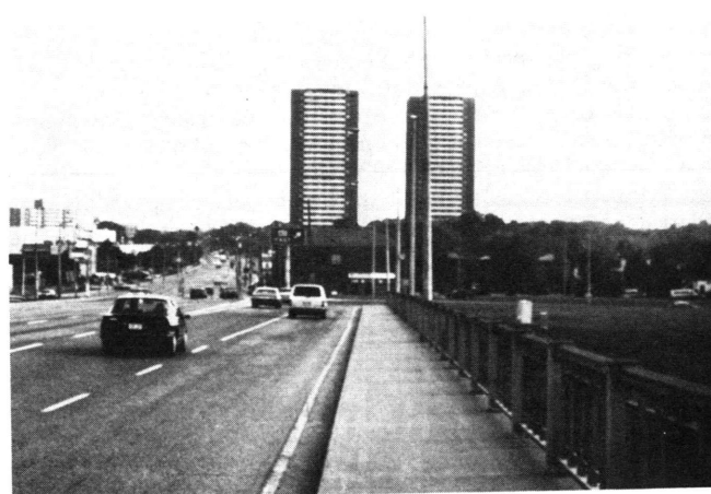
FIGURE 2 Two arterial lanes approach exit to loop ramp (Toronto).
