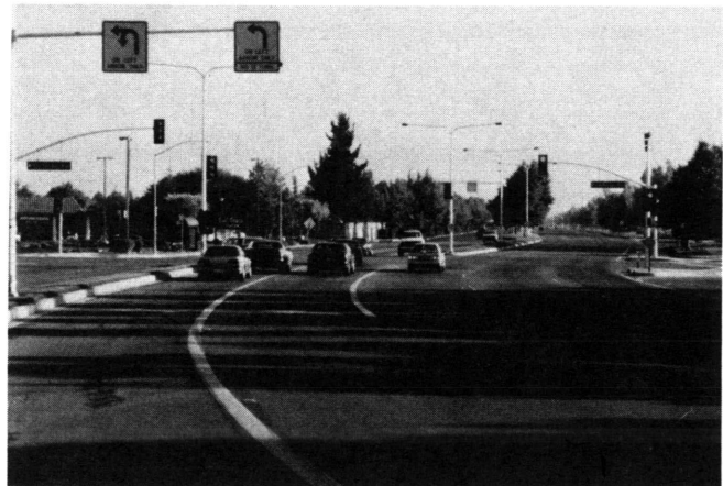
FIGURE 9 Allowing U-turns at low signalized intersections where the cross street has relatively low approach volumes (arterial-collector intersections) facilitates access to properties fronting on major street without the provision of median breaks. A 30-ft median is desirable for such designs. This provides for two turn lanes and a median nose of at least 6 ft.
