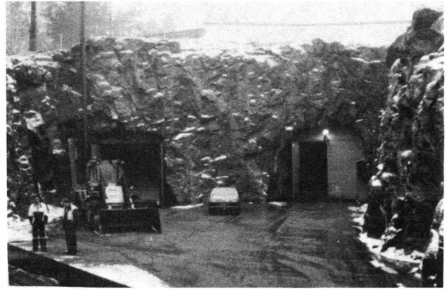
FIGURE 20 Material storage in a rock including sand, granular salt, and mixing unit for brine. Storage is filled from upper level.
