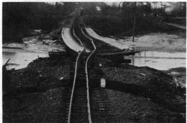
FIGURE 6 The Alaska railroad bridge at Milepost 63.0 that was compressed by lateral ground displacement, causing near end of the bridge to shear connections with the bulkhead and skew to the right [after McCulloch and Bonilla (4)].
