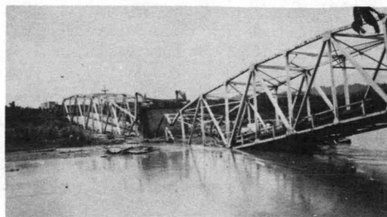
FIGURE 12 Highway bridge that collapsed into the Rio Estrella during the 1991 Costa Rica earthquake (photograph by T. L. Youd).
