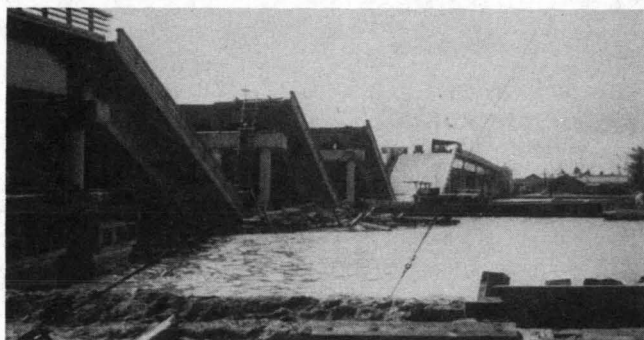
FIGURE 8 Showa highway bridge that collapsed into the Shinano River during the 1964 Niigata, Japan, earthquake (photograph by T. L. Youd).
