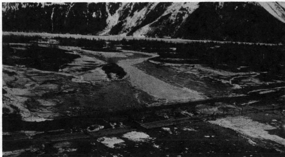
FIGURE 7 Collapsed highway bridge across Twentymile River (bridge nearest camera); a damaged but intact railway bridge is behind highway structure [after McCulloch and Bonilla (4)].
