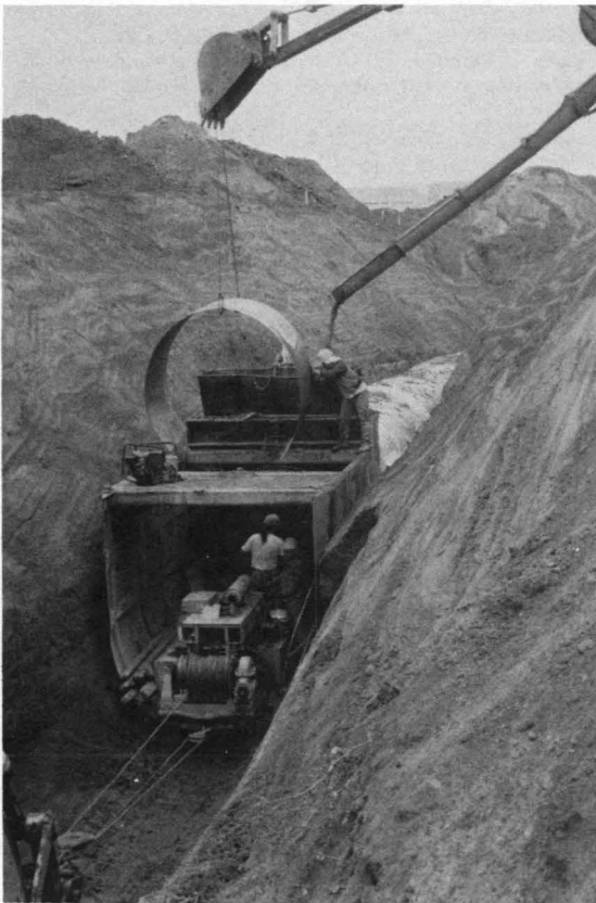
FIGURE 3 Pipe case in prepared trench.
