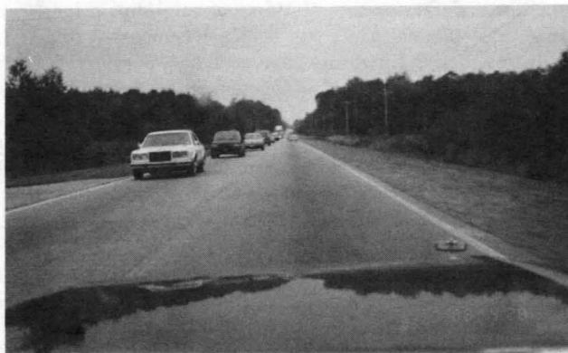
FIGURE 3 Top , Cumbahee River Bridge, US-17, South Carolina. Bottom , US-17 at Green Pond, South Carolina.
