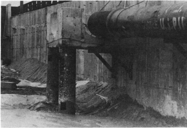
FIGURE 7 Utility placement (I).
