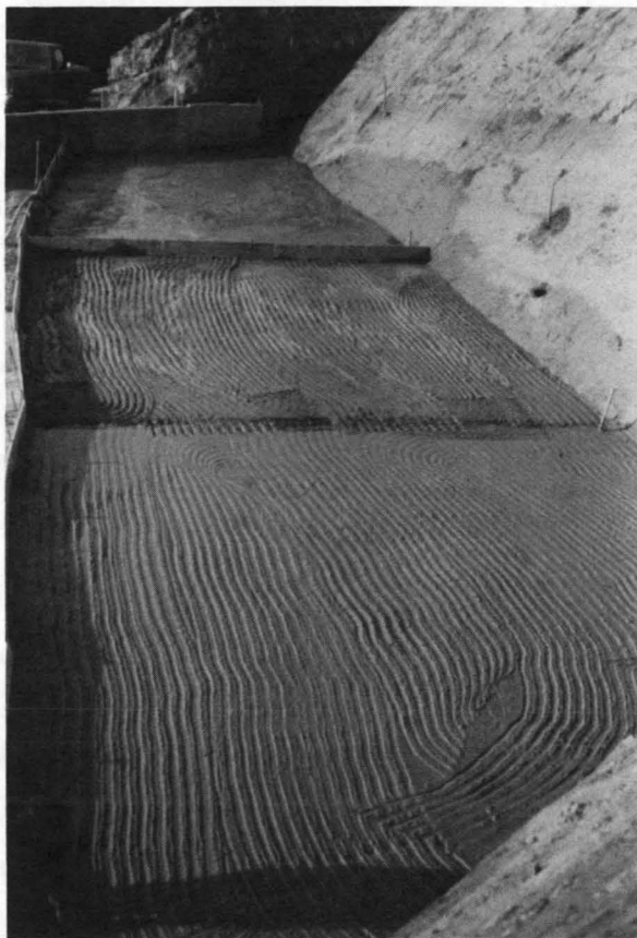
FIGURE 5 Scarified surface of lift (2).
