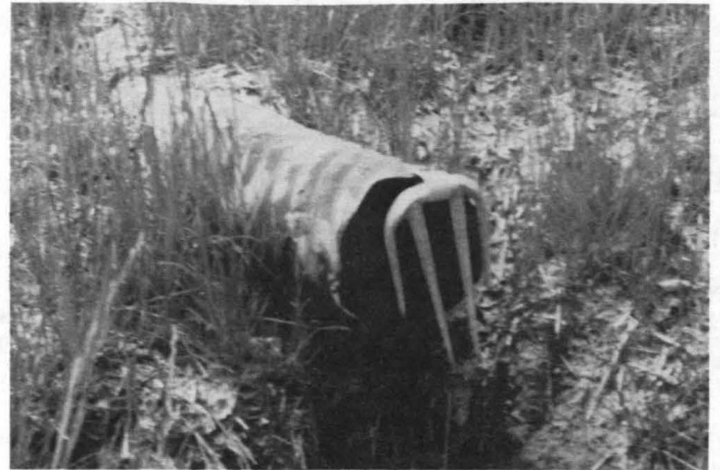
FIGURE 8 Spear-type rodent screen.
