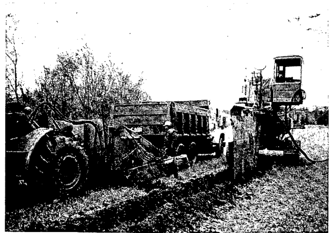
FIGURE 4 Dynapac trenching machine, truck delivering filter aggregate, and shouldering attachment on front-end loader, which places filter aggregate into trench.
