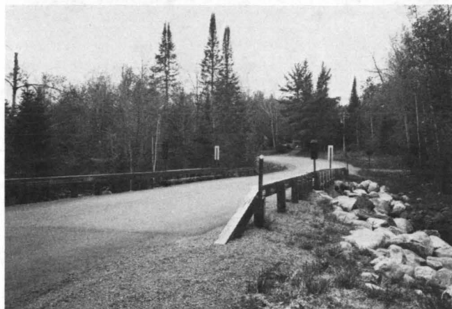
FIGURE 3 Completed Teal River bridge.
