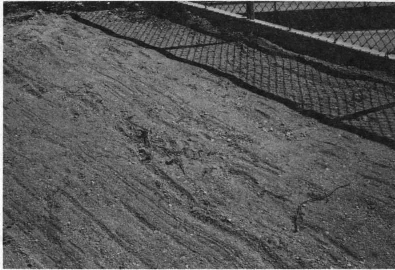
FIGURE 5 Ground surface at excavation site of SR2 geogrid sample.
