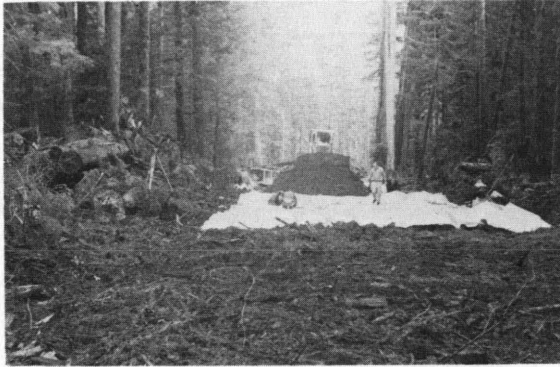
FIGURE 4 Dozer spreading rockfill on geotextile.
