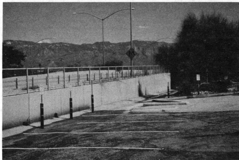
FIGURE 4 Type A wall where SR2 geogrid sample was exhumed.
