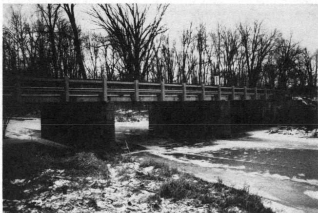
FIGURE 1 Overview of Bridge 1.
