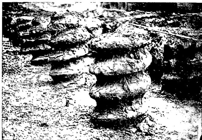
FIGURE 1 Exposed Atlas screw pile.
