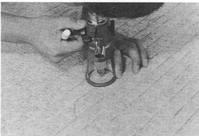
FIGURE 1 Crack width measurement with a measuring microscope.
