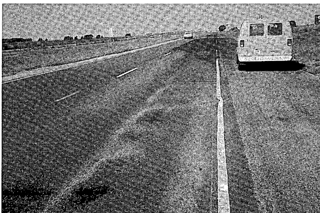
FIGURE 3 Slow traffic lane showing three stages of stripping.
