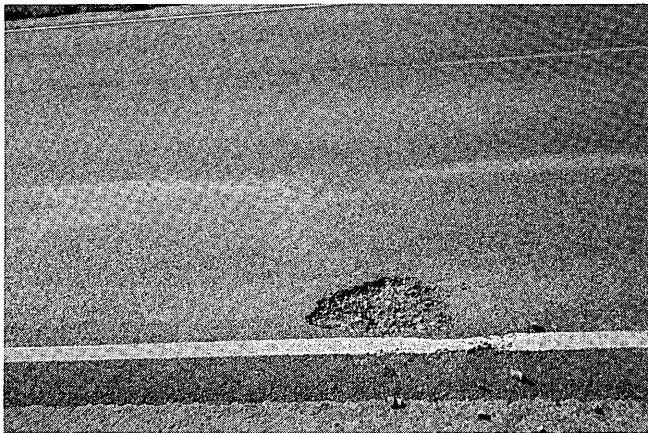
FIGURE 2 Three stages of stripping: white spots, fatty area, and pothole (close up).
