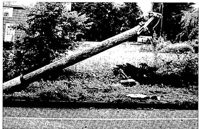
FIGURE 10 Field installation after collision.
