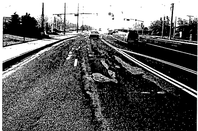
FIGURE 3 Six-month-old pavement that disintegrated.
