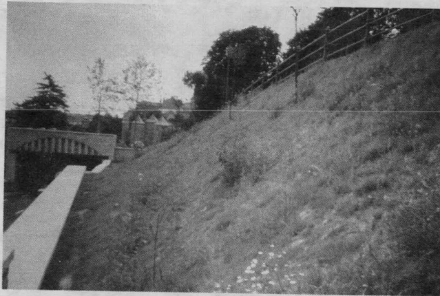
FIGURE 10 (a) Schematic of green method of Texsol production; (b) typical construction site using Texsol green method.
