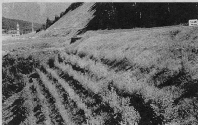
FIGURE 7 Brush-layer embankment fill stabilization after 2 years showing grass and brush establishment (Brenner Pass highway, Austria).
