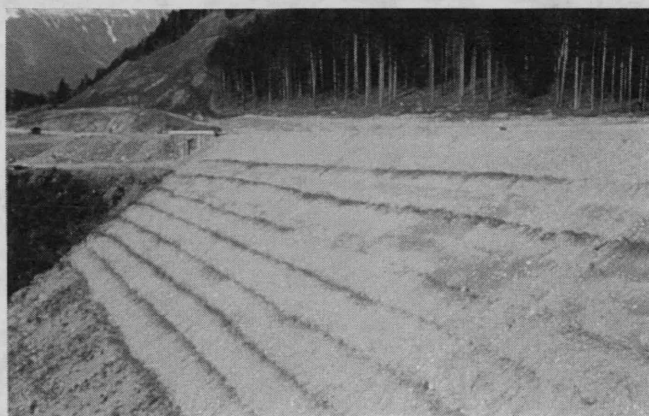
FIGURE 6 Brush-layer embankment fill stabilization immediately after construction (Brenner Pass highway, Austria).
