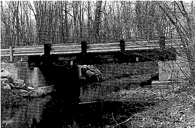
FIGURE 5 Side view of bridge.
