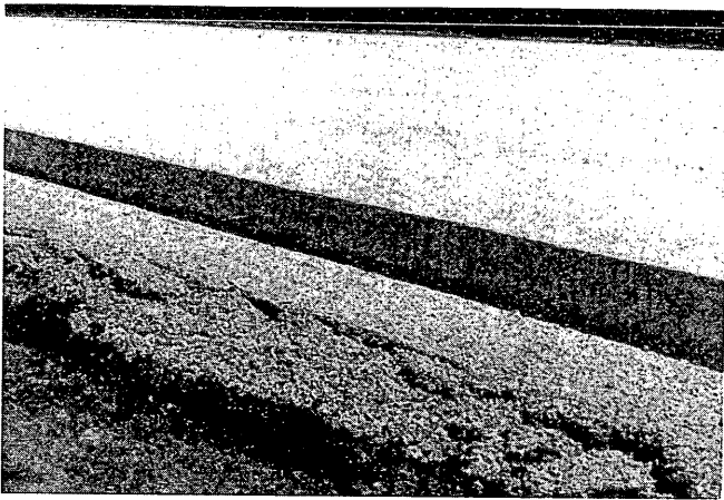
FIGURE 11 Broken OGD.
