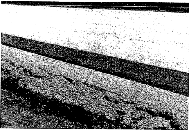
FIGURE 11 Broken OGD.
