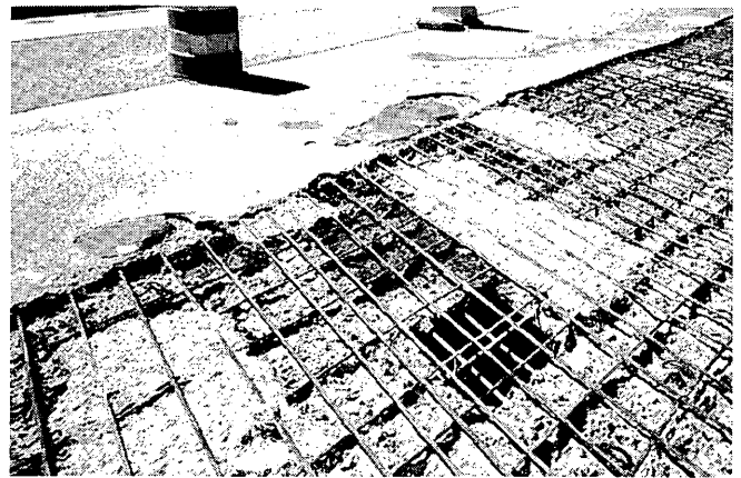
FIGURE 3 Existing patches on a hydrodemolished bridge deck.
