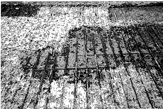
FIGURE 1 Hydrodemolished bridge deck surface.
