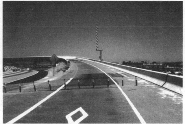
FIGURE 7 Entrance ramp to HOV. This is northbound entrance from State Highway 163. It indicates hydraulic pop-ups and barrier gate. At this time, HOV facility is closed. When access is allowed in this direction, pop-ups are down. When HOV is open in opposite direction, pop-ups are up and gate is down.
