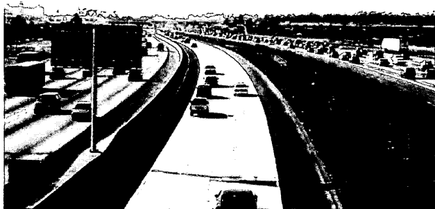
FIGURE 4 HOV during operation. Reversible HOV facility in median. Northbound traffic Level of Service (LOS) F at p.m. peak period near southerly entrance.
