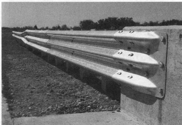
FIGURE 2 Triple T installation for Tests 19 and 20.
