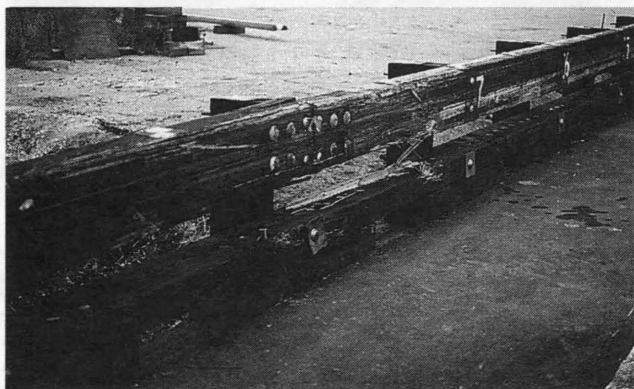
FIGURE 7 Impact location, vehicle damage, and bridge rail damage, Test FSCR-4.
