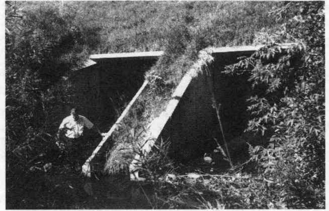
FIGURE 10 View of inlet end of concrete box culvert.
