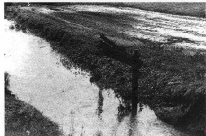
c. FAILED TIE-DOWN SYSTEM.
