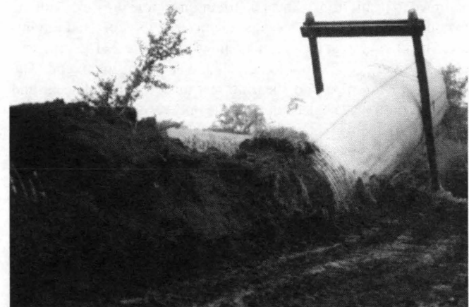
b. PULL-OUT OF TIE-DOWN SYSTEM.
