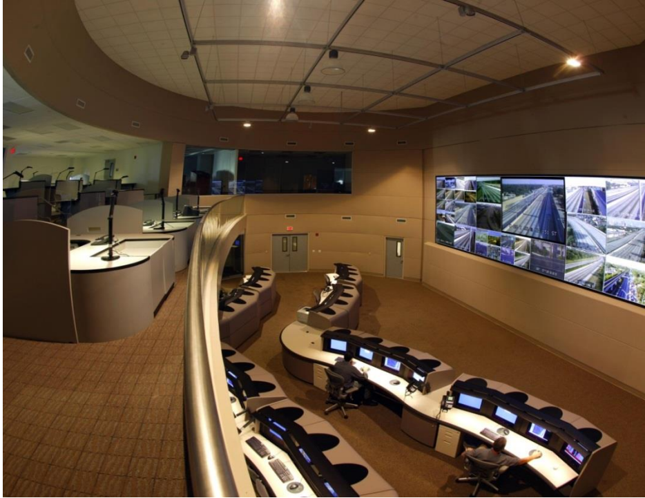
Original layout of the FDOT D6 RTMC.
