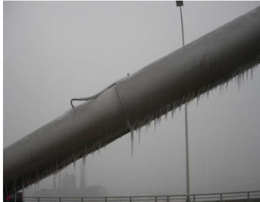
Ice accumulation on the east side of VGCS (2011)
