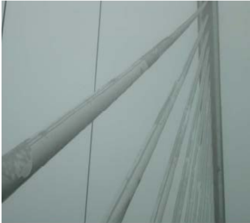
Ice accumulation pattern on VGCS stays (2011)
