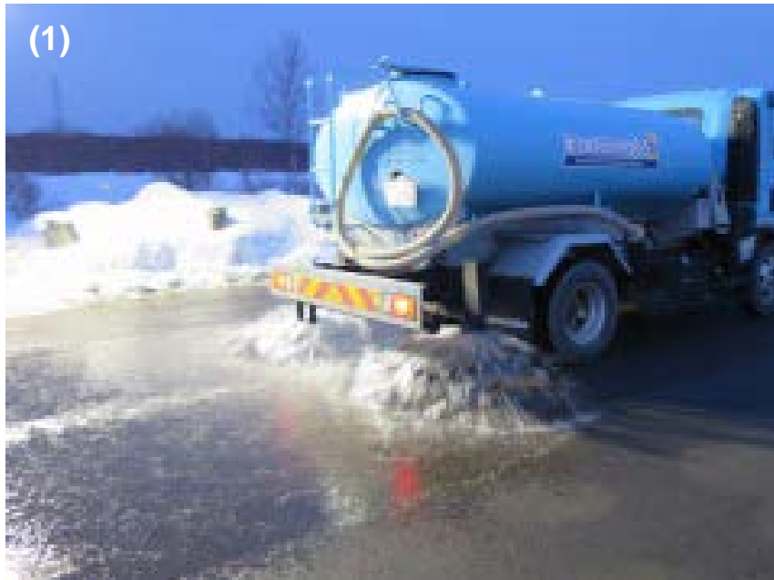
Sprinkling water for making ice film on the surface
