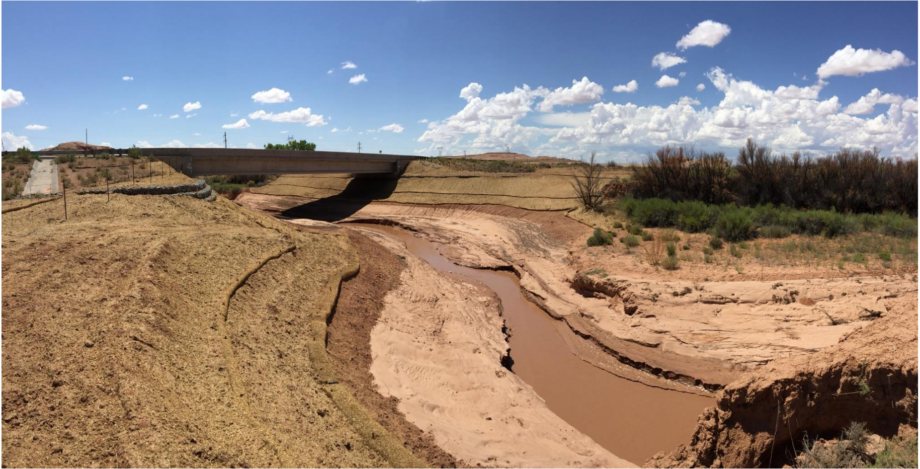
November 2017 – State Route 160 Laguna Creek Bridge (Final grading and seeding)
