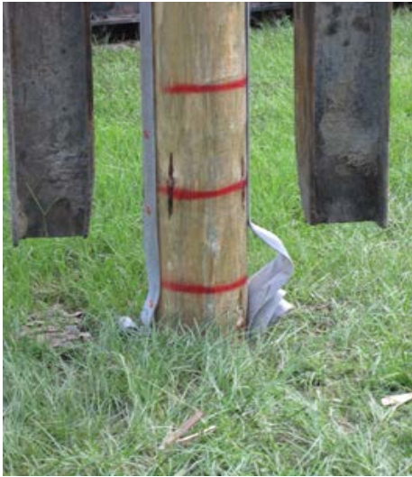
FIGURE 3.3 First pile prototype during installation during buckling of PVD.
