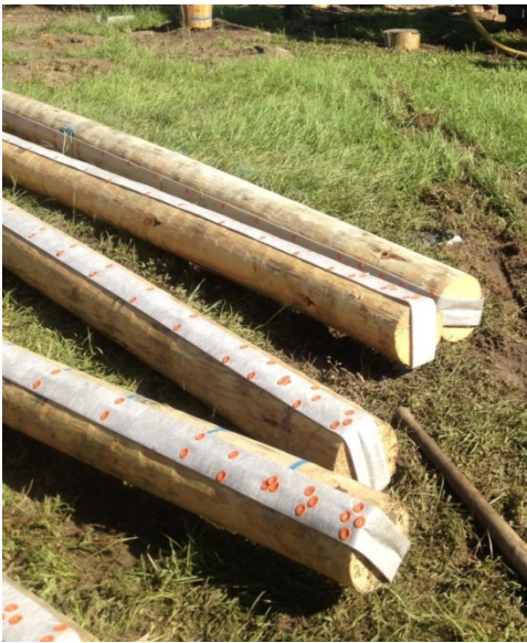
FIGURE 3.5 Second pile prototype with additional fasteners.
