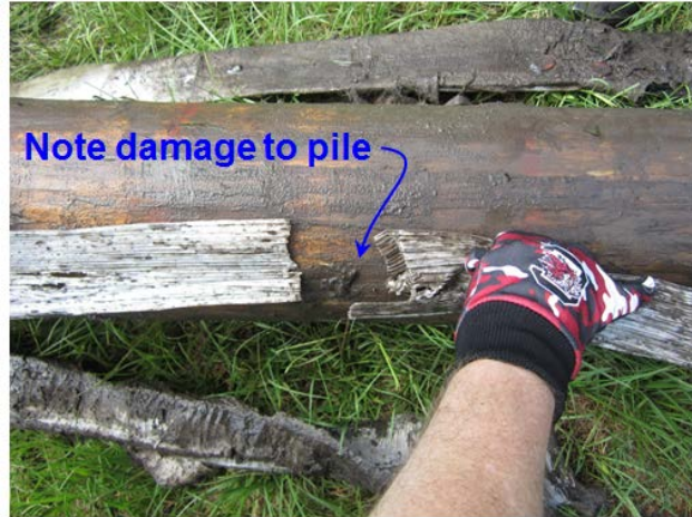
FIGURE 3.4 Damaged PVD and timber pile prototype.
