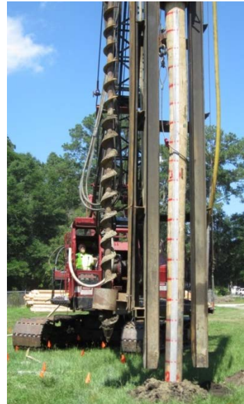
FIGURE 3.6 Installation of second pile prototype within pre-drilled cavity.
