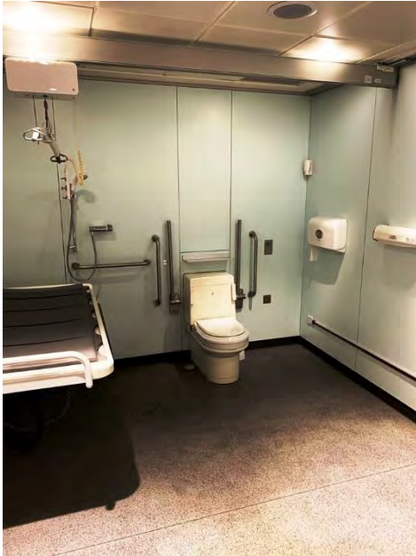
CHANGE TABLE RESTROOM Change table and toilet. Hoist above.
