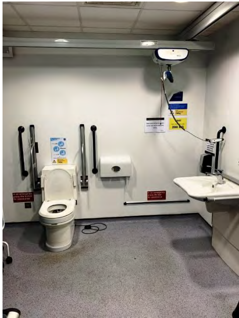
CHANGE TABLE RESTROOM - Toilet and adjustable height lavatory
