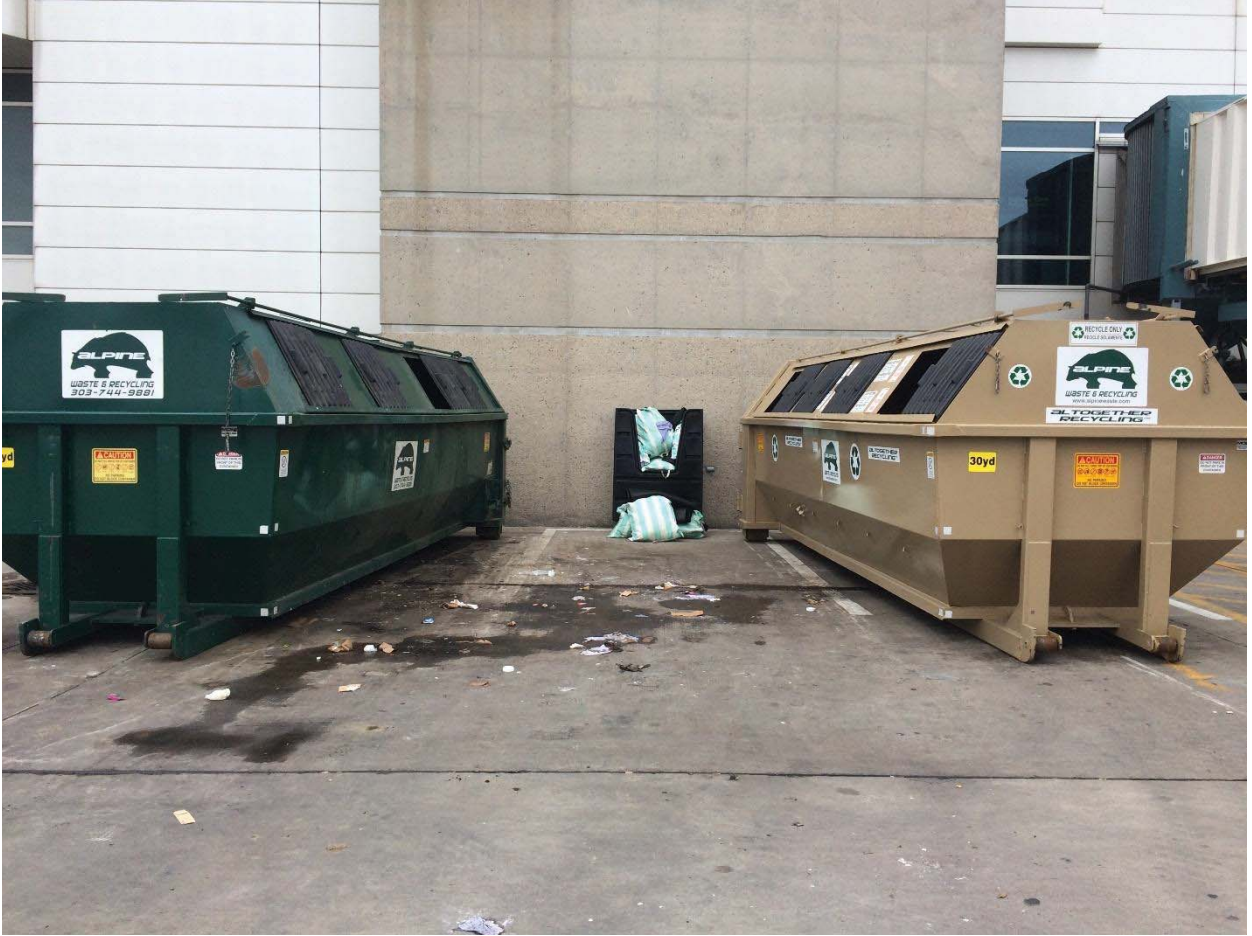
Figure 5: Ramp level waste and recycling front load roll-off dumpsters, courtesy of Denver International Airport
