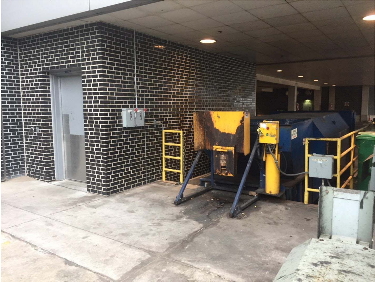
Figure 1: Entrance to compost container wash facility, courtesy of Metropolitan Airports Commission
