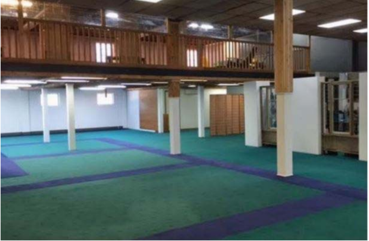
Figure 5: Removed carpet reinstalled as flooring; courtesy of Port of Portland
