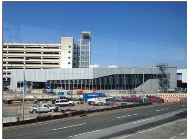
Terminal F Baggage Claim Building Under Construction
