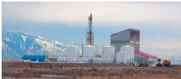
Glycol Plant at SLC
