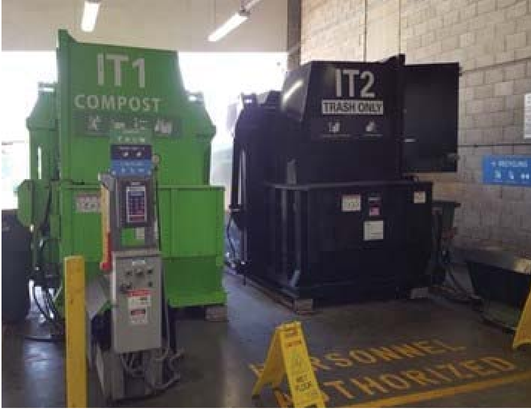
Standard signage on Materials Recovery Area compactors; courtesy of San Francisco International Airport
