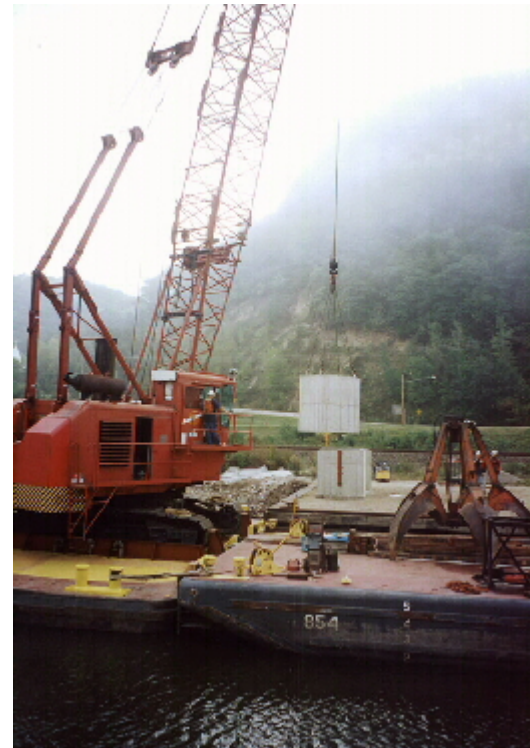
USACE crane barge helps with gage building replacement at L&D 8
