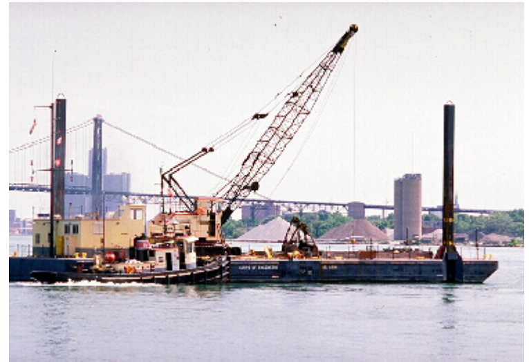
USACE crane barge on the Detroit River.
