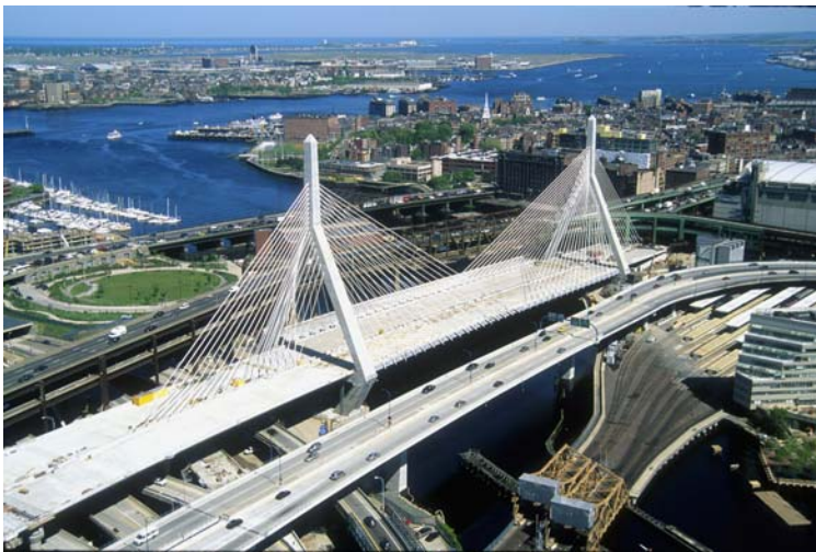
Leonard P. Zakim Bunker Hill Bridge, Boston Photo courtesy of Central Artery/Tunnel Project
