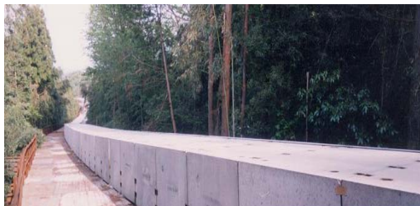
(c) PCP outside the tunnel for waste transport
