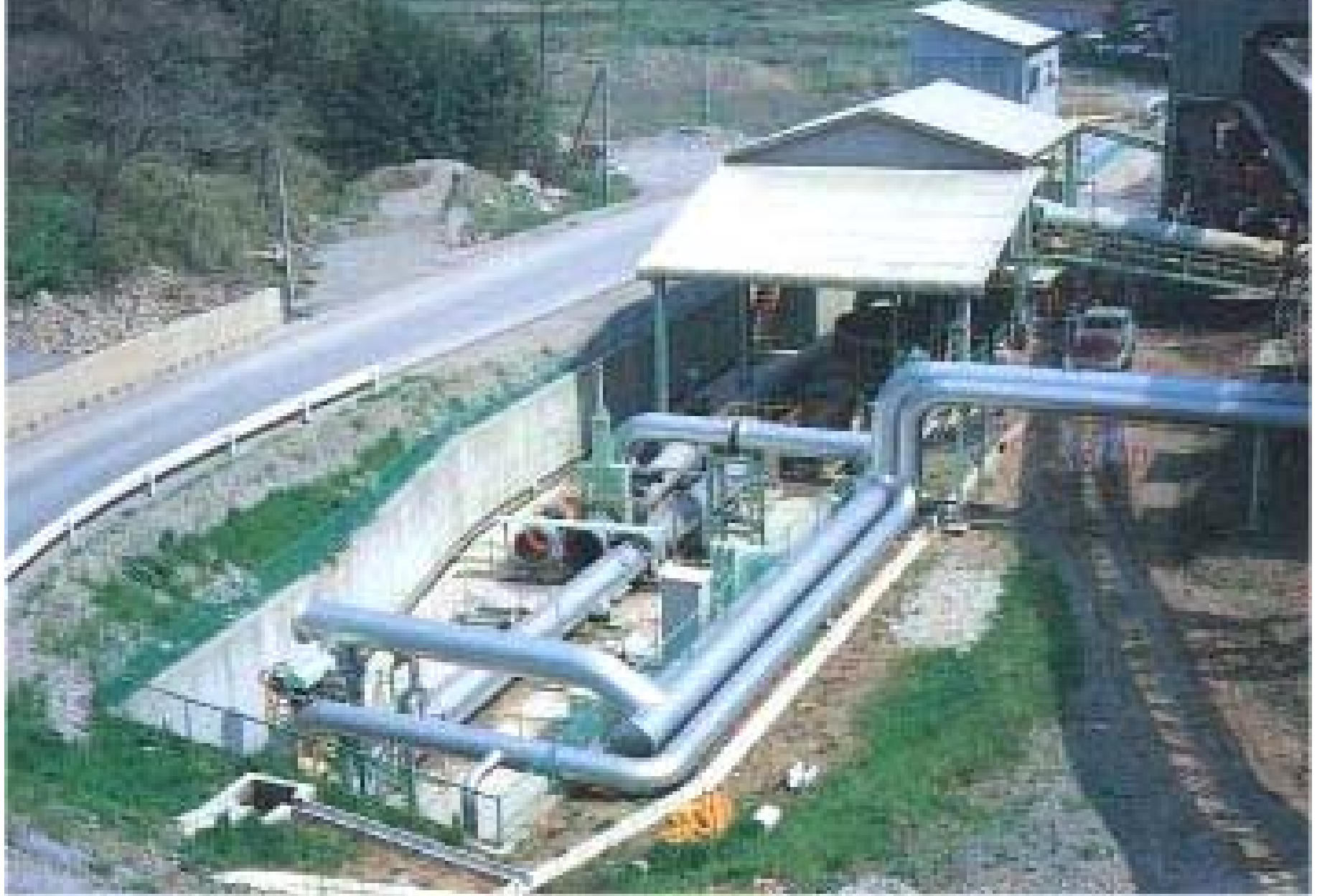
The intake of PCP in Kuzuu, Japan for limestone transport
