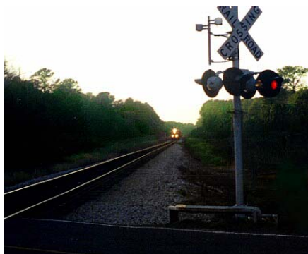
Figure 6. The above photograph shows the system installation at the KCS site with the south looking sensors installed.
