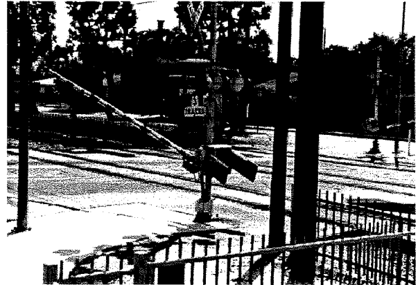
Figure 5-2. Quad gate crossing metal structures.
