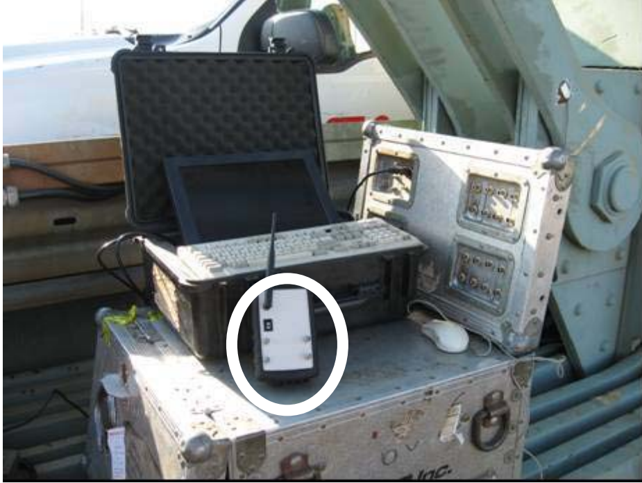
FIGURE 1 Wired and wireless systems shown on CN's Victoria Bridge in Montreal. The wireless system is shown circled on the metal box that houses the wired system's PC. Shown on top of the metal box are the monitor and keyboard which are required to setup and run the wired system.
