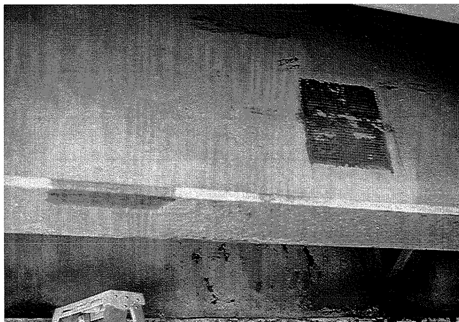
FIGURE 14 Results of tests at Pucketa Creek bridge. Removed ElectroPad™. One-square-foot test and wrap-around test.
