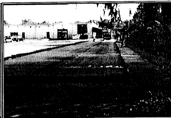
Figure 4. One of 5 PQI Test Strips
