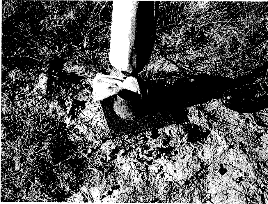
Figure 71 Photograph of an EQ Drain tied to an anchor. Anchors measured 150 mm x 150 mm x 12.5 mm. Generally, the anchors had the corners bent over; this
