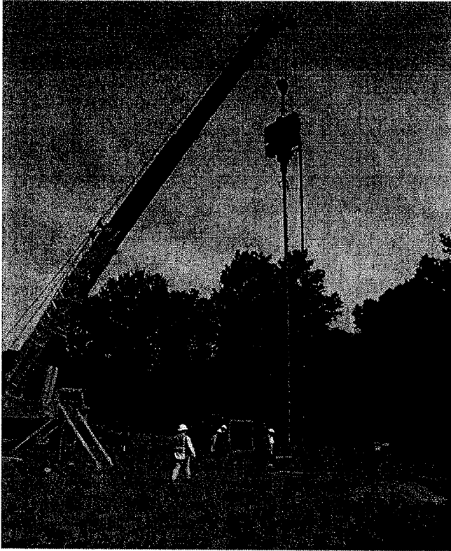
Figure 69 Drain installation was accomplished with the use of a 70 ton crane and a vibratory hammer and mandrel.
